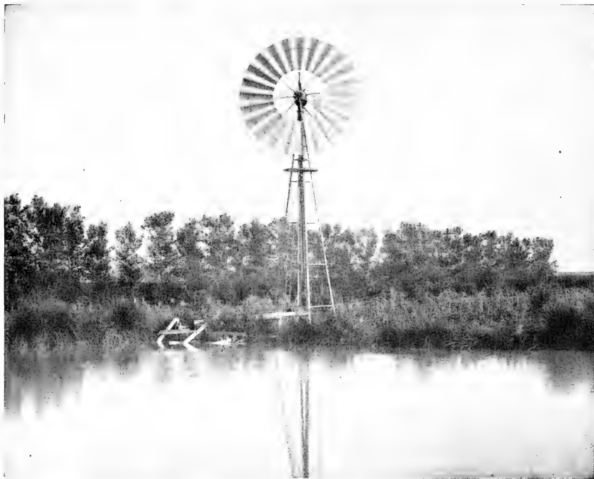
TYPICAL WINDMILL AND RESERVOIR FOR IRRIGATION.
